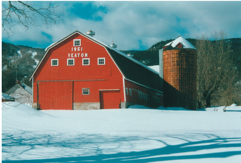
Cover Photograph by: John C. Porter, Boscawen, N.H., The Yeaton Barn was built in 1951, and has been used over the years to house heifers and cows that were bought and sold as part of a cattle dealer business. A three-bag cement mixer was used to pour the entire foundation, which has been subject to frost heaving due to poor drainage. Dean Yeaton has recently improved the drainage around the foundation and put new metal roofs on all the buildings to preserve them. The barn is located on Yeaton Road, off Route 25 in Plymouth, N.H.
